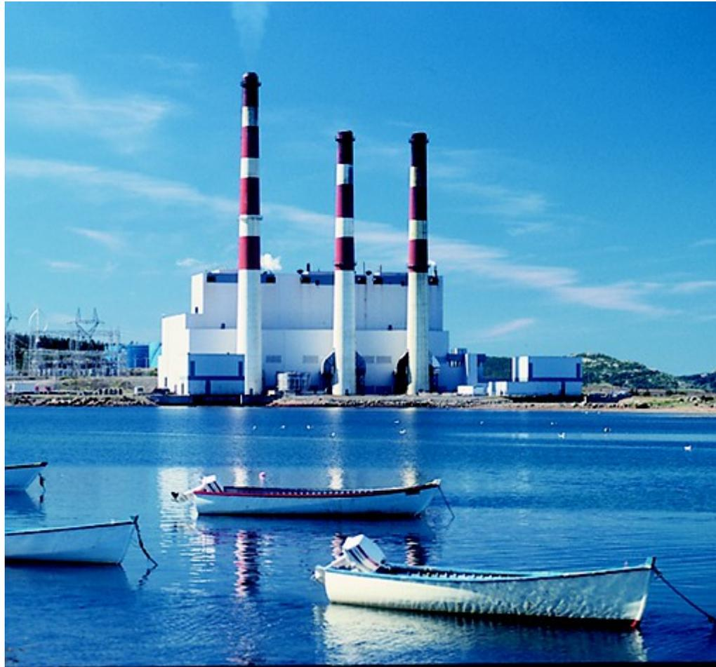
The (***Holyrood***) plant was constructed in two stages. In 1969, Stage I, consisting of two generating units (Units 1 and 2) each capable of producing 150 MW, was started and placed in service in April 1971. In December 1979, Stage II, consisting of one generating unit (Unit 3) capable of producing 150 MW, was completed.
